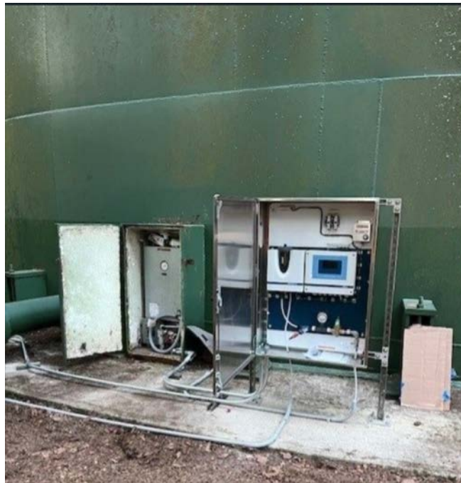
New RTU Water Quality Panel
