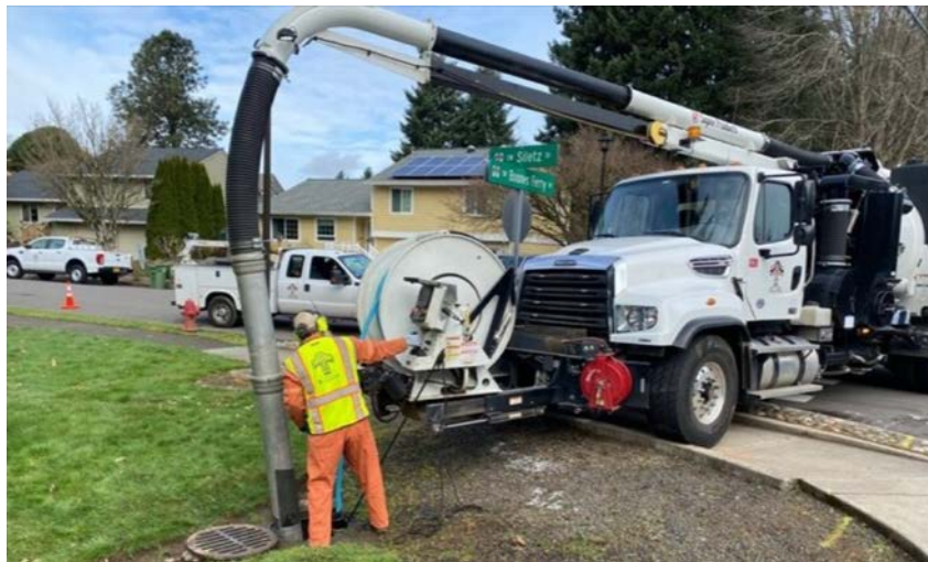
Storm System Cleaning
