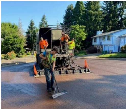
Slurry seal roadway
