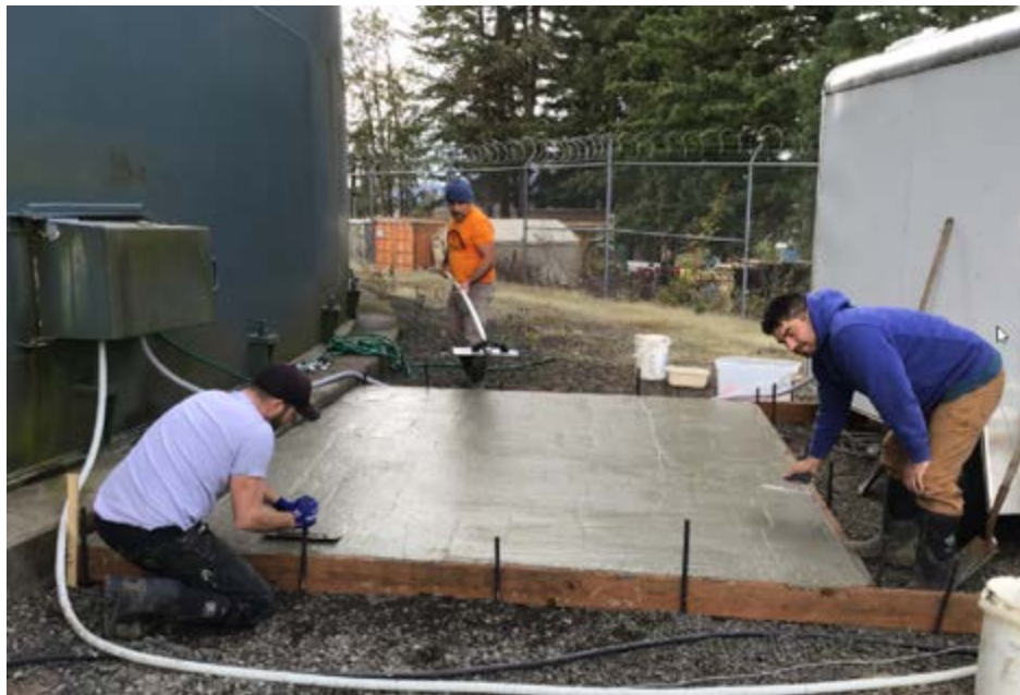
Pouring concrete at water reservoir
