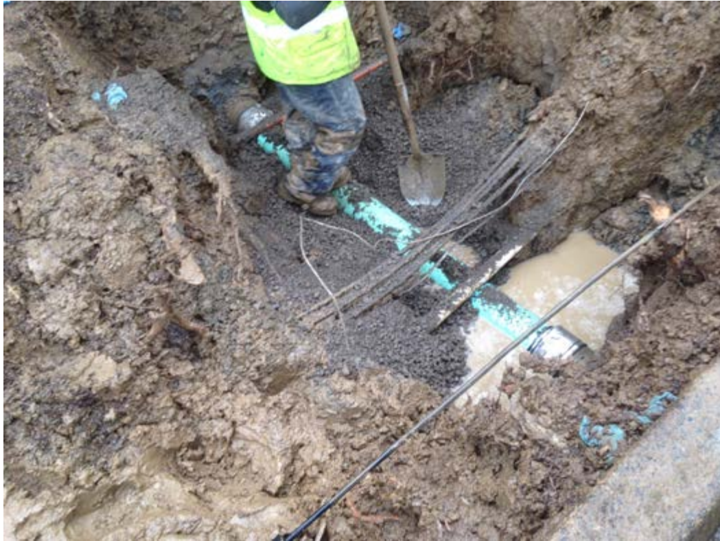
Sewer Lateral Repair
