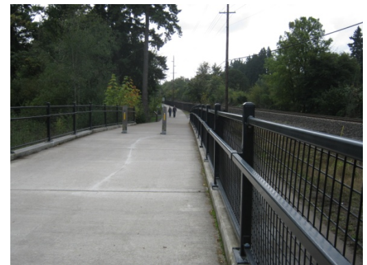
Concrete path in Tualatin Community Park
