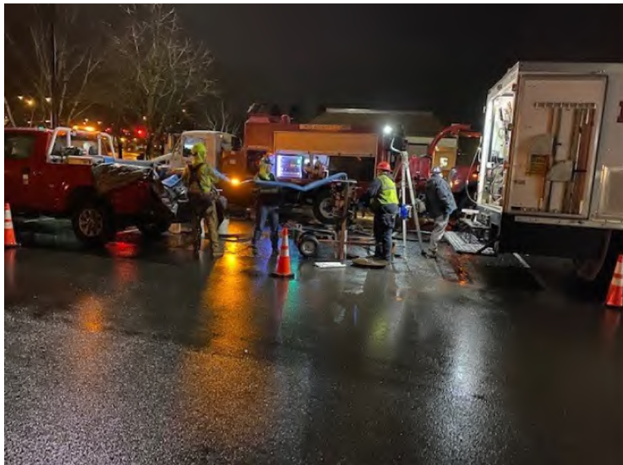
Sewer Main Line Repair
