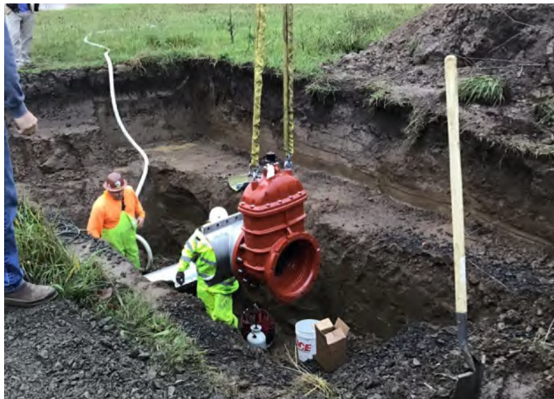
Installing a gate valve
