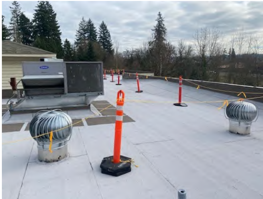
Juanita Pohl Center Roof Project
